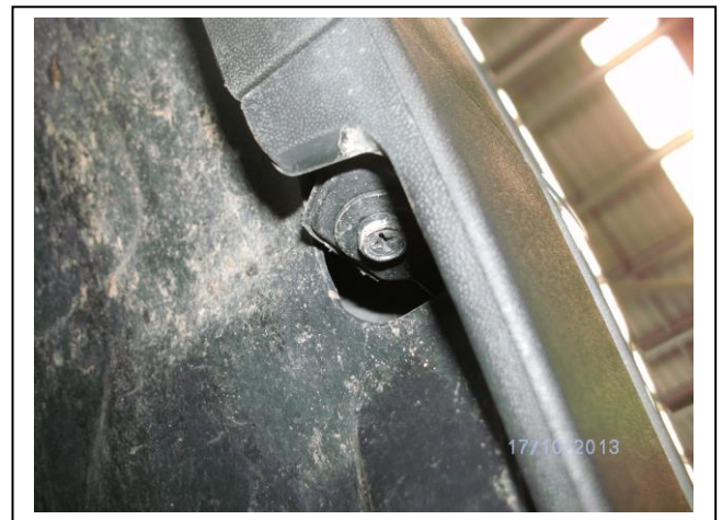
Figure 2: Bolt in rear of plastic bumper
